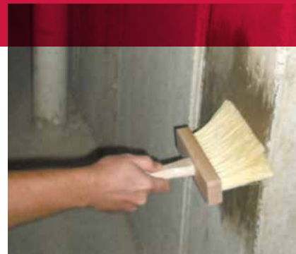
Applying waterproofing material with a masonry brush.
