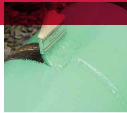
Applying pipe coating to weld seams.
