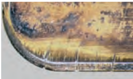
Small cracks at 90° with reference to cutting edge
