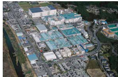
Sendai Facility (JAPAN)
