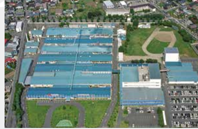
Okaya Facility (JAPAN)
