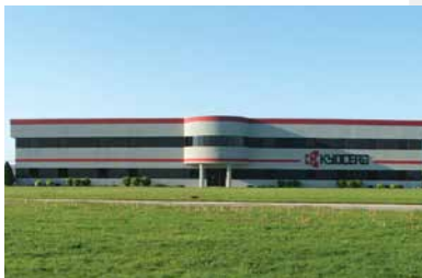
Ohio Facility (USA)
