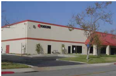
California Facility (USA)
