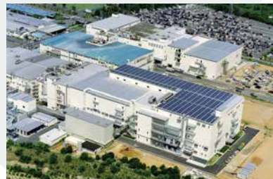
Yokaichi Facility (JAPAN)
