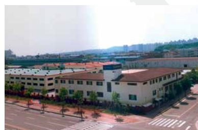
Incheon Facility (KOREA)
