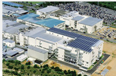
Yokaichi Facility (JAPAN)
