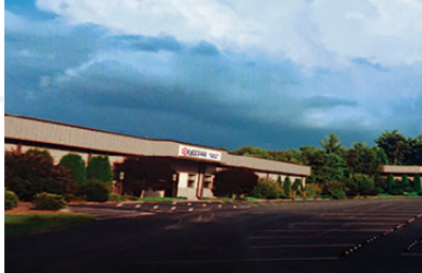
North Carolina Facility (USA)
