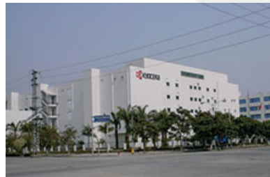
Silong Facility (CHINA)
