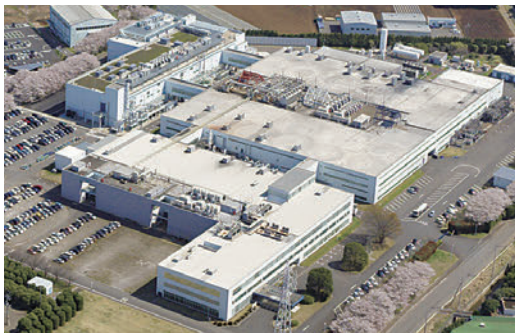
MITSUBISHI MATERIALS CORPORATION TSUKUBA PLANT (JAPAN)
