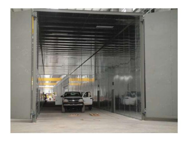
Interior shot – New design using galvanized wall and roof panels instead of painting all sheets.
