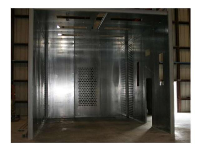
Exhaust plenum in rear wall, paint exhaust plenums in the rear/side corners. Paint exhaust fan will mount on the roof of the booth for a straight thru the roof stack. Paint filter cover doors not yet installed.
