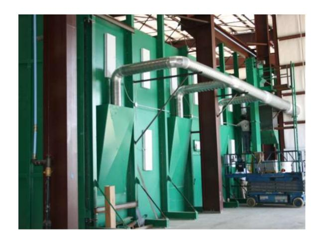
Right side of booth – (6) exhaust plenums attached to dust collector
