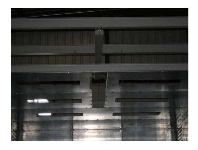
10' slot seal for overhead hoist.
