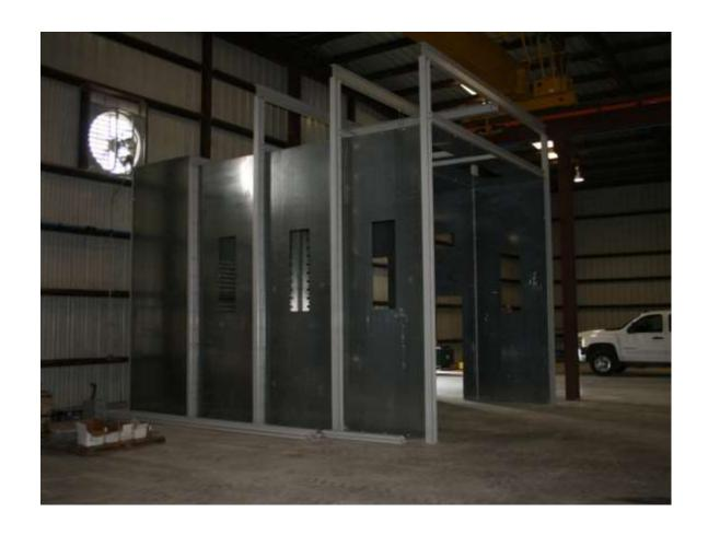
Additional structural steel for 2 ton hoist.
