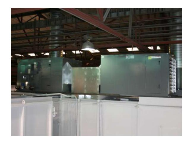
Two heated air make-up units. These can be used independent or together to heat for ambient or cure cycle.
