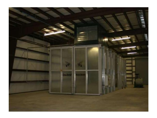
20,000 CFM heated air make-up unit mounted on the roof of the booth.
