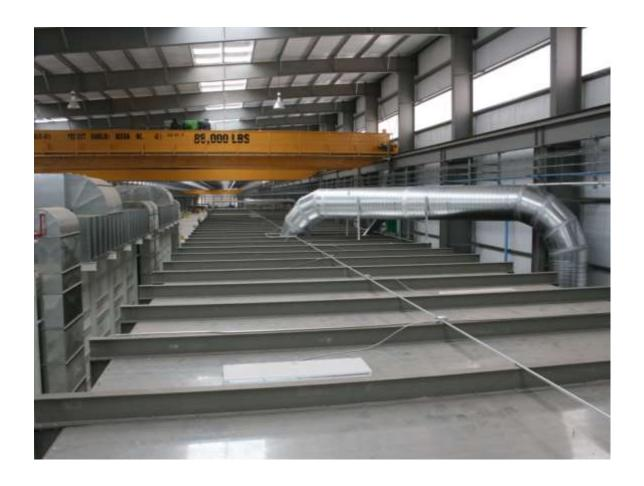
Roof view – ducting in foreground is for the dust collector. Ducting at the far end (booth entrance) is for a metalizing collector system.
