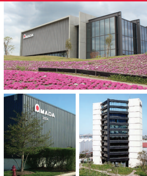
top: TOKI PLANT; bottom right: ISEHARA HQ; bottom left: U.S. MAIN OFFICE IN SCHAUMBURG, IL
