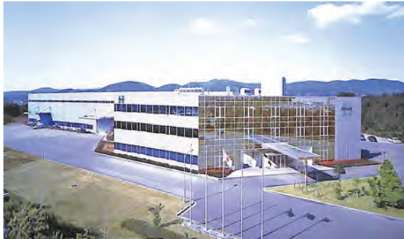
Heian Miyakoda system research center located in Shizouka, Japan.
