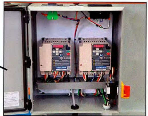
Electrical enclosure with variable frequency drive. 3 phase 230/460 volts NFPA-79 specifications 24 VDC control circuit Overload protected
