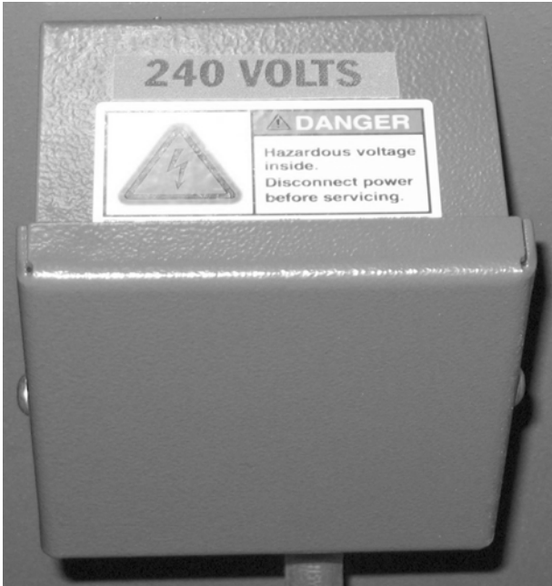
Power Junction Box
