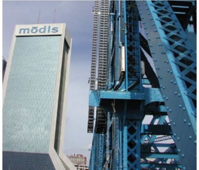
Nylatrac Modular TL carriers, with anodized aluminum crossbars for added strength in heavy wind conditions, maintain the lines for electric and hydraulic controls on a vertical lift bridge.
