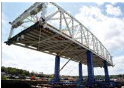
Incremental bridge lifting
