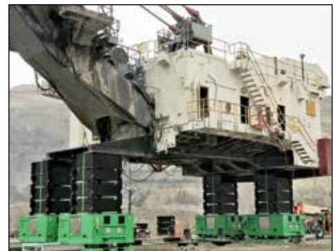
▼ Undecking an 1500-ton Electric Rope Shovel in a Copper Mine with a JS500 Jack-Up System for bearing inspection and maintenance.
