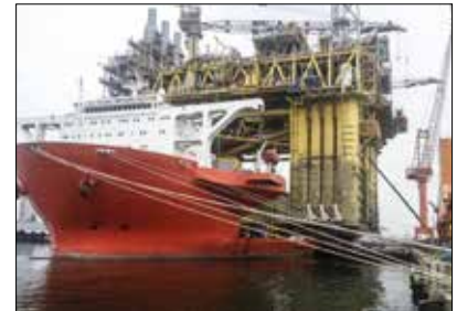
Synchronous superlift and launch
