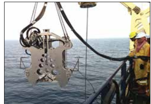
▲ MDWS Diamond Wire Saw lowered into sea.
