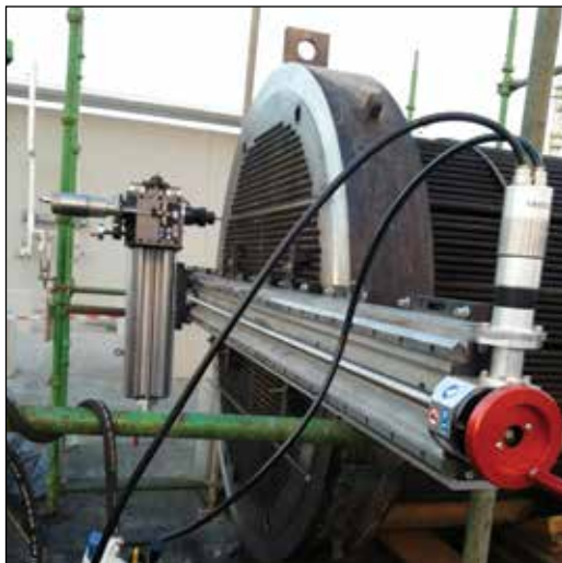
▼ MRY Milling machine on a heat exchanger.
