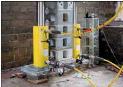
Bridge lifting and launching
