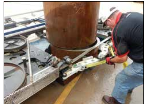
▲ Pipe cutting with BS portable band saw.
