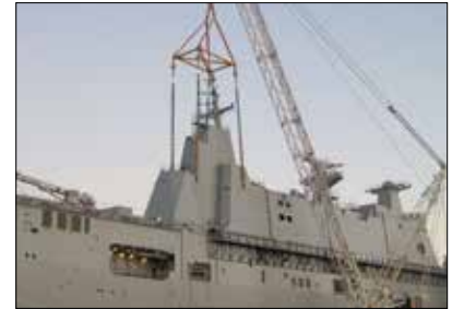
Synchronous hoisting and load positioning
