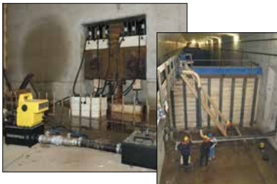
◀ Enerpac lightweight aluminum RAC506 cylinders are ideal for wet environments such as this tunnel under the river (Holland High-Speed Train Line).
