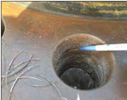
▲ A typical thread before refurbishment
