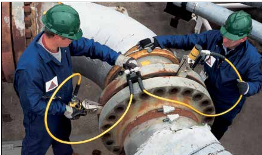
◀ Two FSH14 spreaders used simultaneously with Enerpac handpump, hoses and AM21 control manifold.
